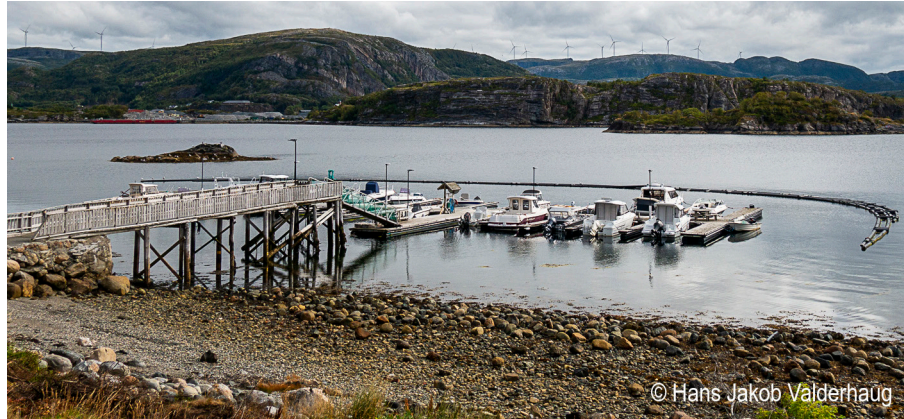
The small pontoon system at Harsvika in Stokksundet.
