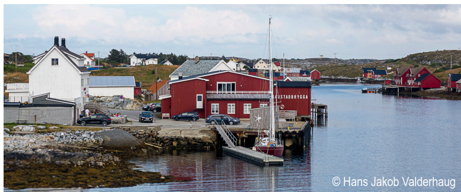
Titran visitors' pontoon, looking east.
