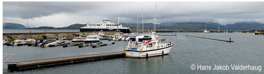
Right: The visitors' pontoon north in the harbour at Brekstad, looking south.
