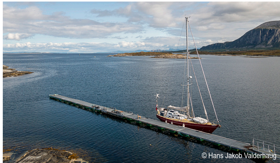
The deep-water visitors' pontoon at Ringholmen, looking northeast.
