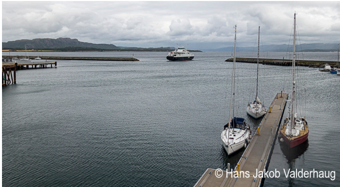
Above: The visitors' pontoon southwest in the harbour at Brekstad, looking southeast.
